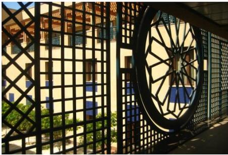
The design of the building was inspired by mashrabiya, which was used as a secrecy element in arabic architecture, shading, ventilation. This structure of Mashrabiya was applied to the structure with strengthened by technology and controlled by the sunlight [24,25].
