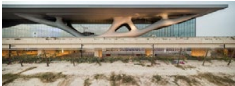
Figure 6. The constructed slab of the Unikabeton project Qatar National Convention Center and its carrier steel pipes [10]
