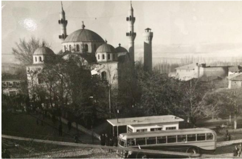
Figure 2. The original state of the structure and the restoration after the 1893 earthquake, where the minaret was left unfinished as a reminder of the earthquake [28].
