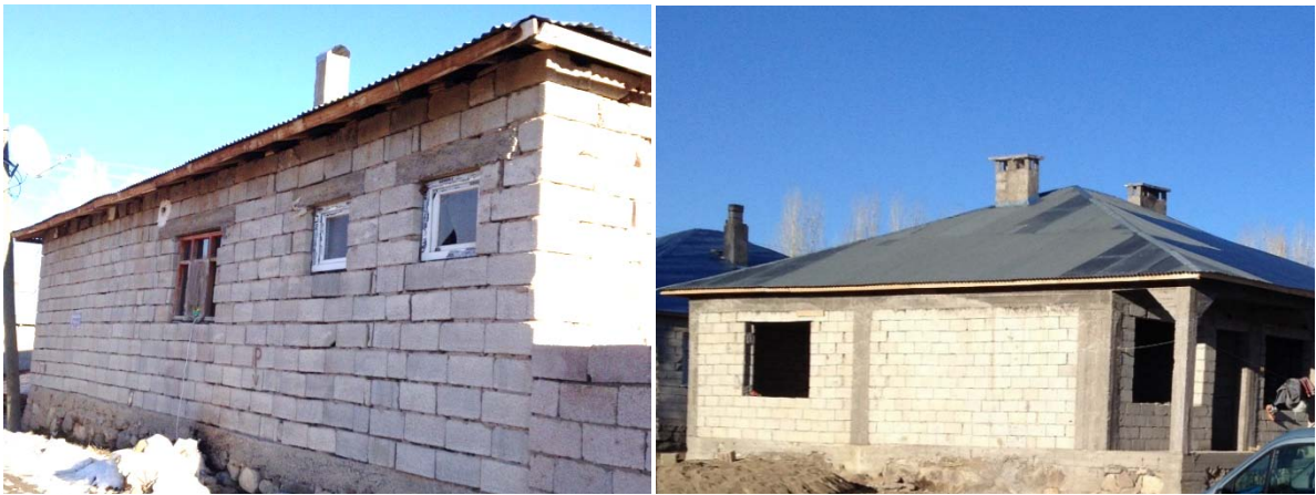
Figure 11. Village of Bayramli / Van/ Application of briquette structure photographed by Hakan Irven
