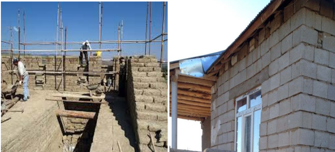
Figure 5. The construction of adobe wall
