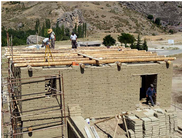
Figure 3. Village of Karahan / Van / Application of wooden roof [4] Figure 4. Village of Bayramli /Van / stone foundation photographed by Hakan Irven
