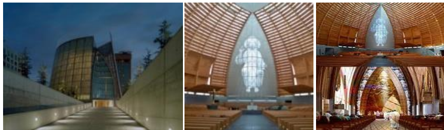
Figure 5. Cathedral of Christ the Light – the cathedral made of wood and glass in Auckland California [URL 6]
