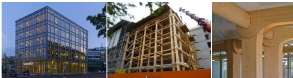
Figure 2. Wooden Headquarters Tamedia in Zurich [URL 2]
